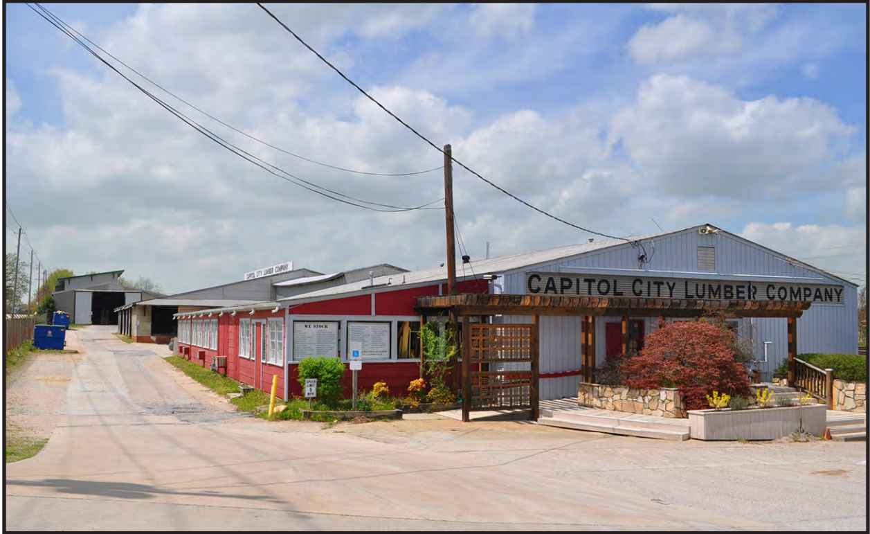
Figure 6. Main Complex, Looking West
