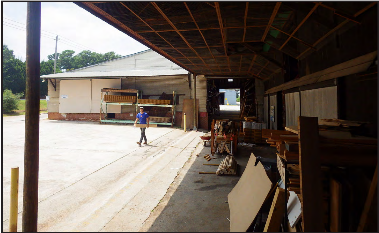
Figure 17. Hardwood Warehouse, East Side
