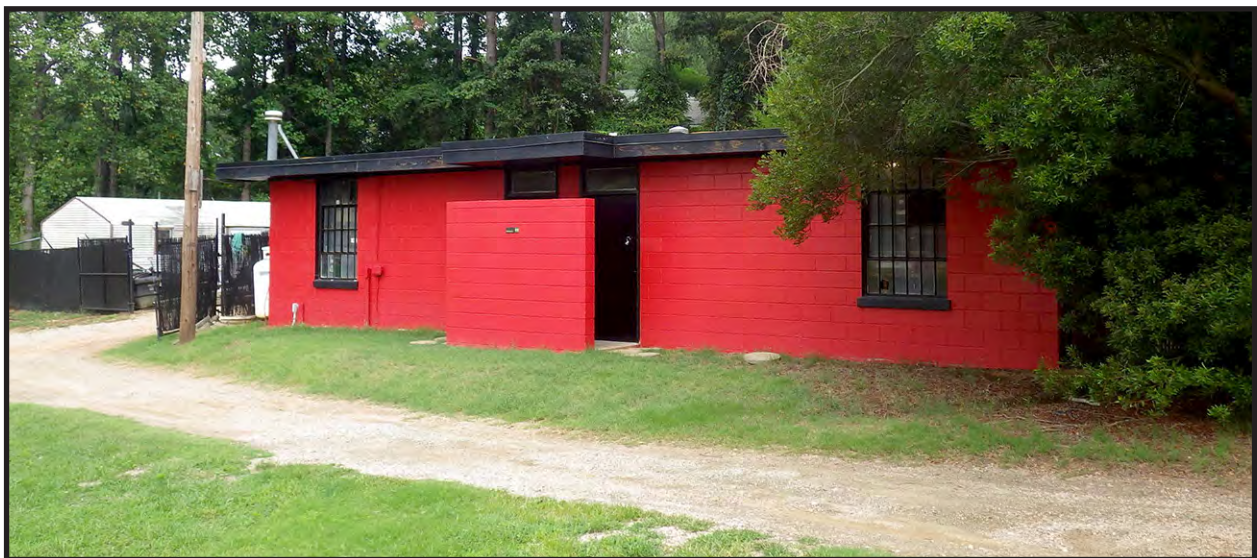
Figure 63. Maintenance Building, West Side
