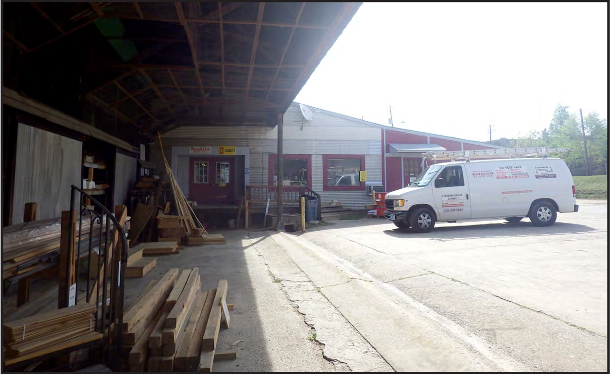
Figure 11. West Side of Hardware Store and Office Addition
