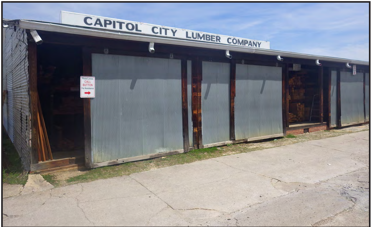
Figure 19. Hardwood Warehouse, South Side Sliding Doors
