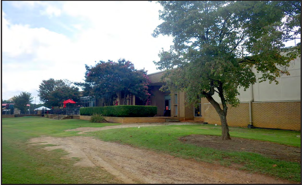
Figure 74. Rear Elevation, Looking East with 2010 Kitchen Wing Right of Frame
