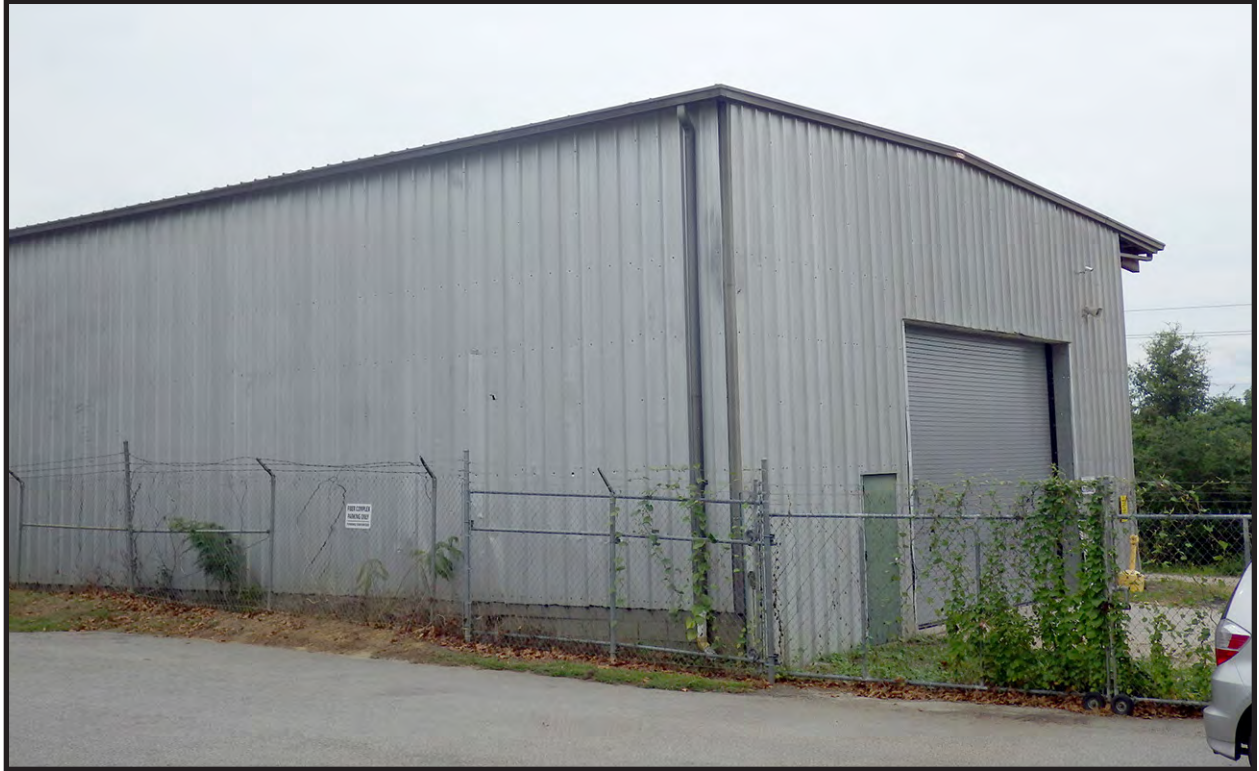
Figure 26. Warehouse #3, South and East Sides
