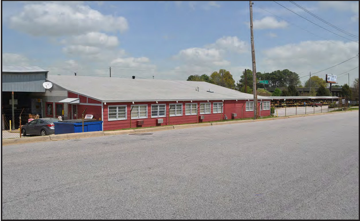
Figure 10. Office Addition, South Side
