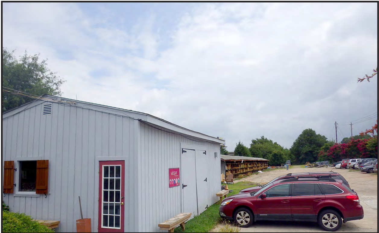
Figure 5. Storage Shed, South and West Sides
