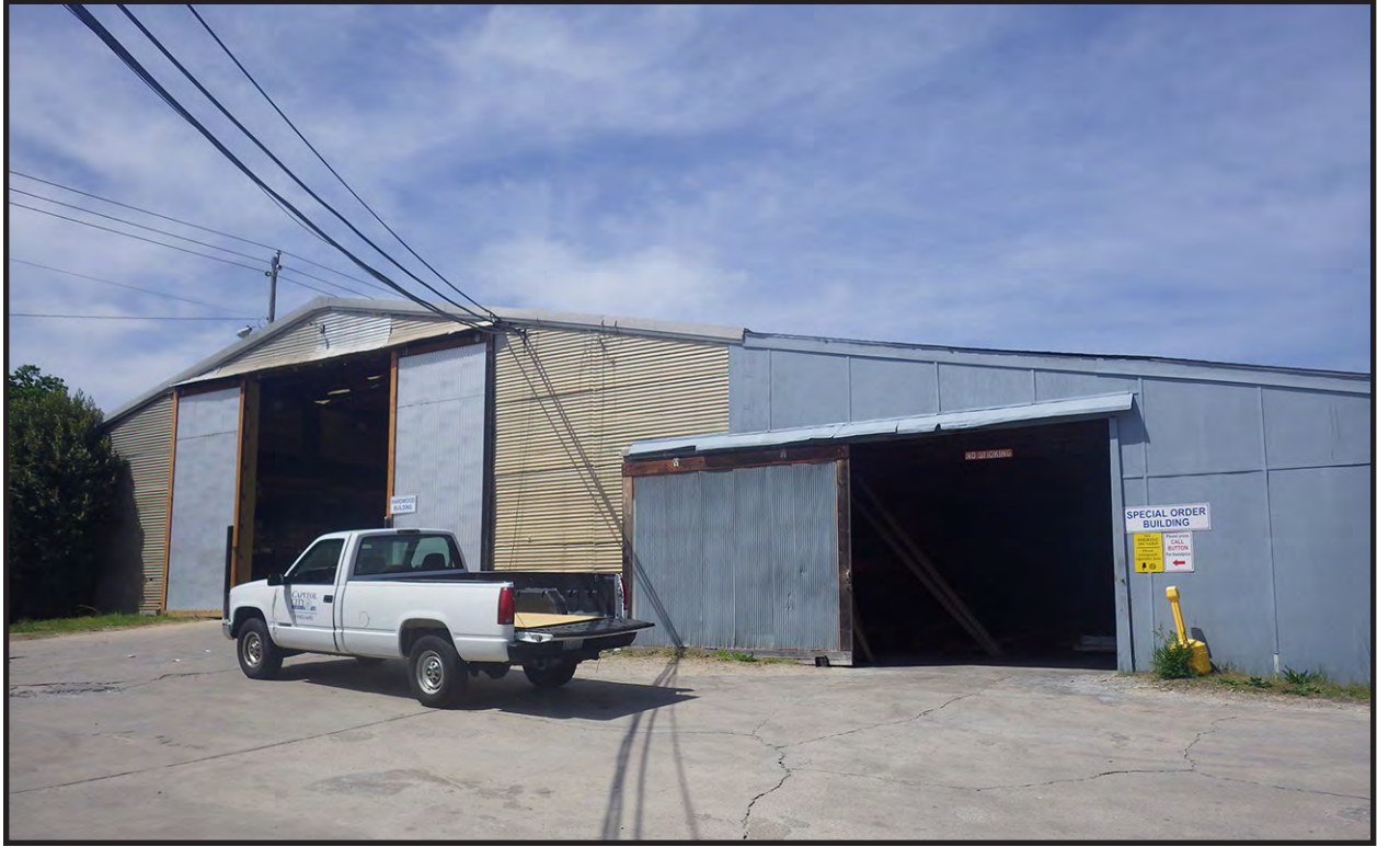
Figure 22. AB Building, East Side
