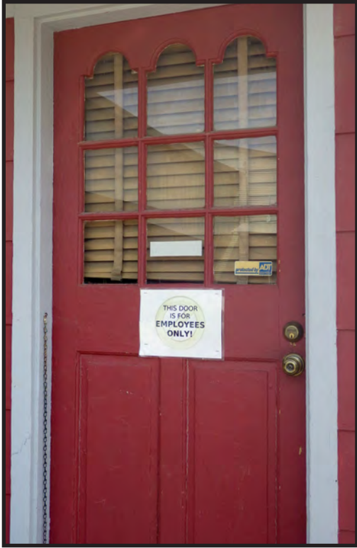
Figure 12. Original Door in West Side of Office Addition
