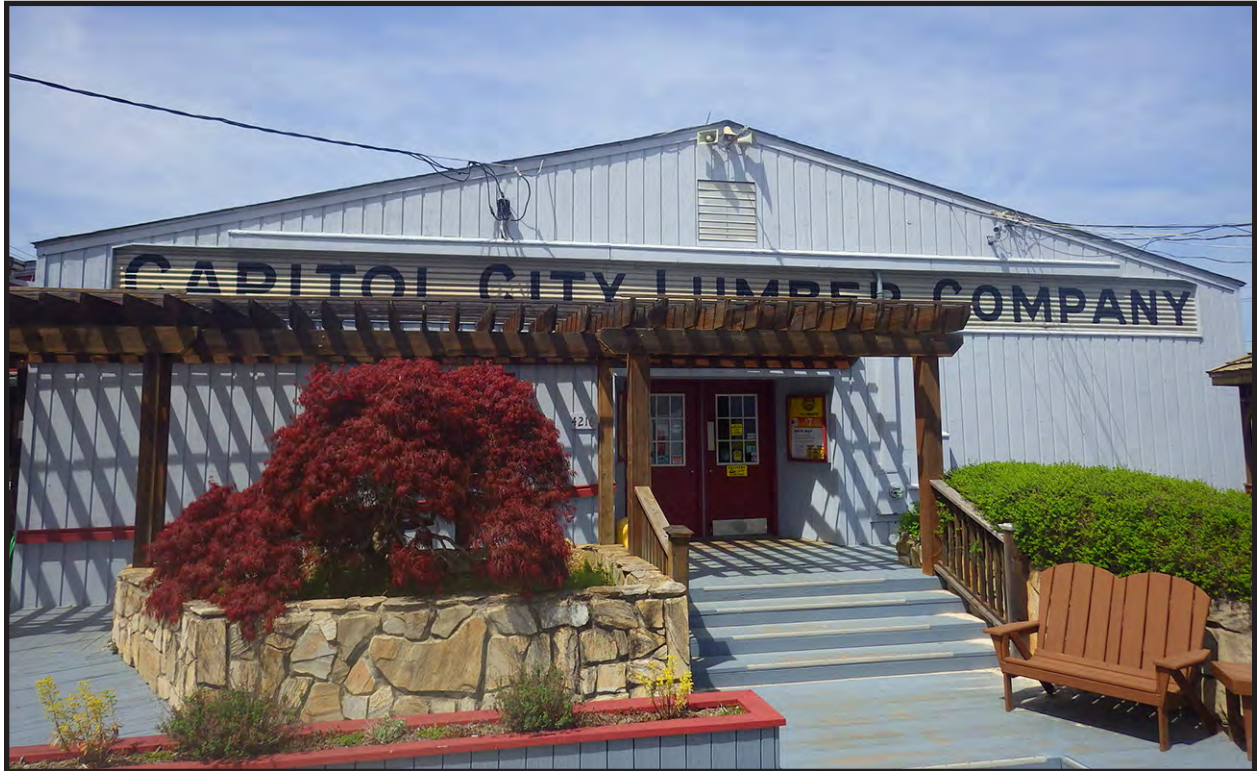
Figure 7. East Side of Hardware Store
