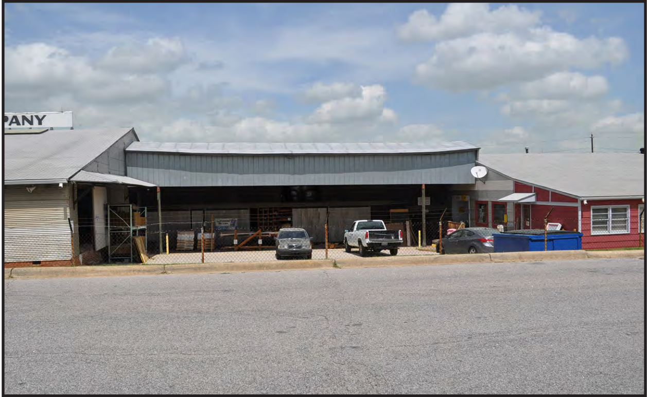
Figure 16. Sawshed, South Side
