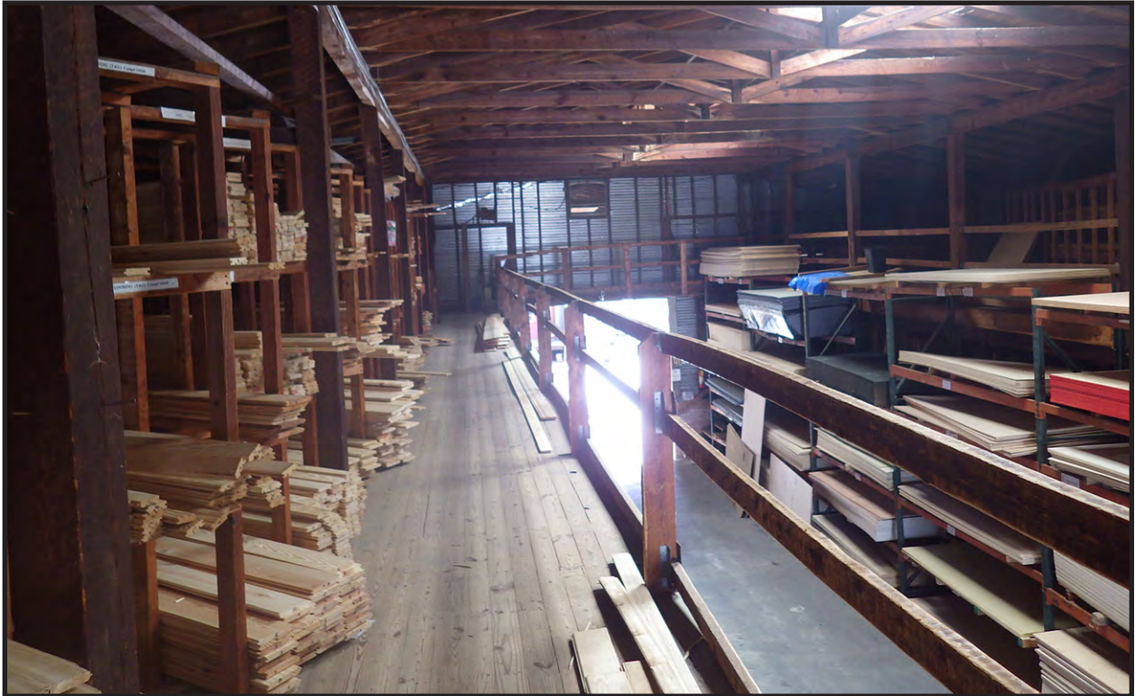
Figure 21. Interior Hardwood Warehouse, Looking West from South Catwalk
