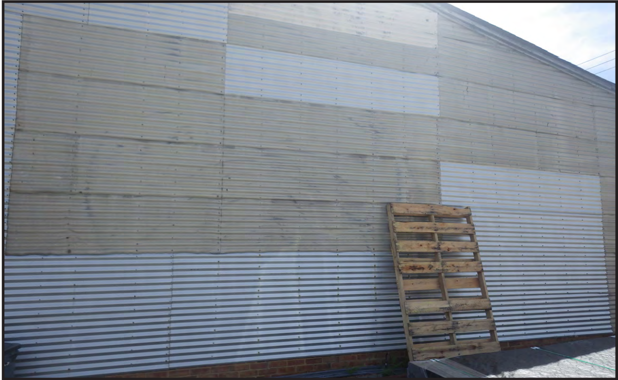
Figure 23. Original and Replacement Siding on West Side of AB Building
