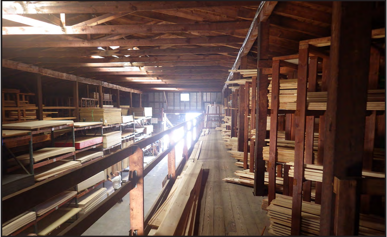
Figure 20. Interior Hardwood Warehouse, Looking West from North Catwalk
