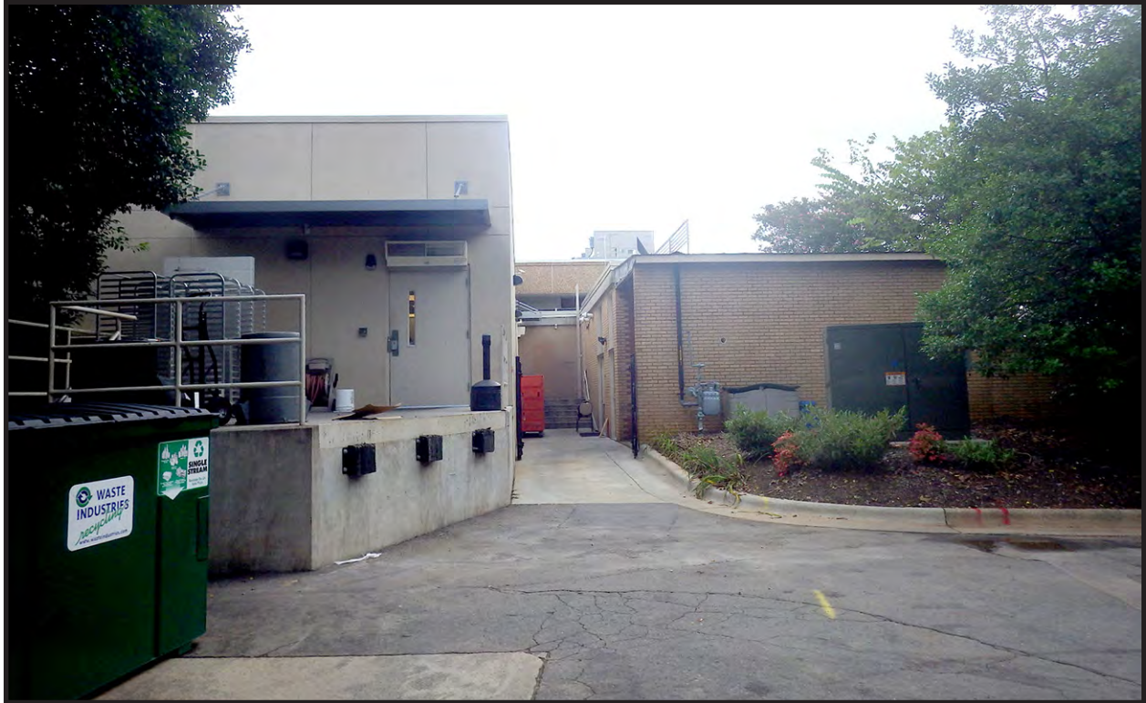
Figure 75. West Side, Showing 2010 Kitchen Wing (Left) and Original Kitchen Wing (Right)
