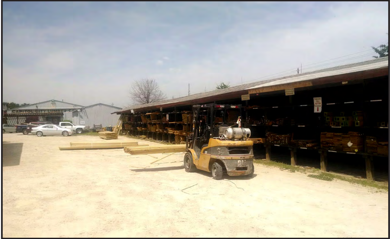
Figure 4. Treated Lumber Storage Shed, Built ca. 1975
