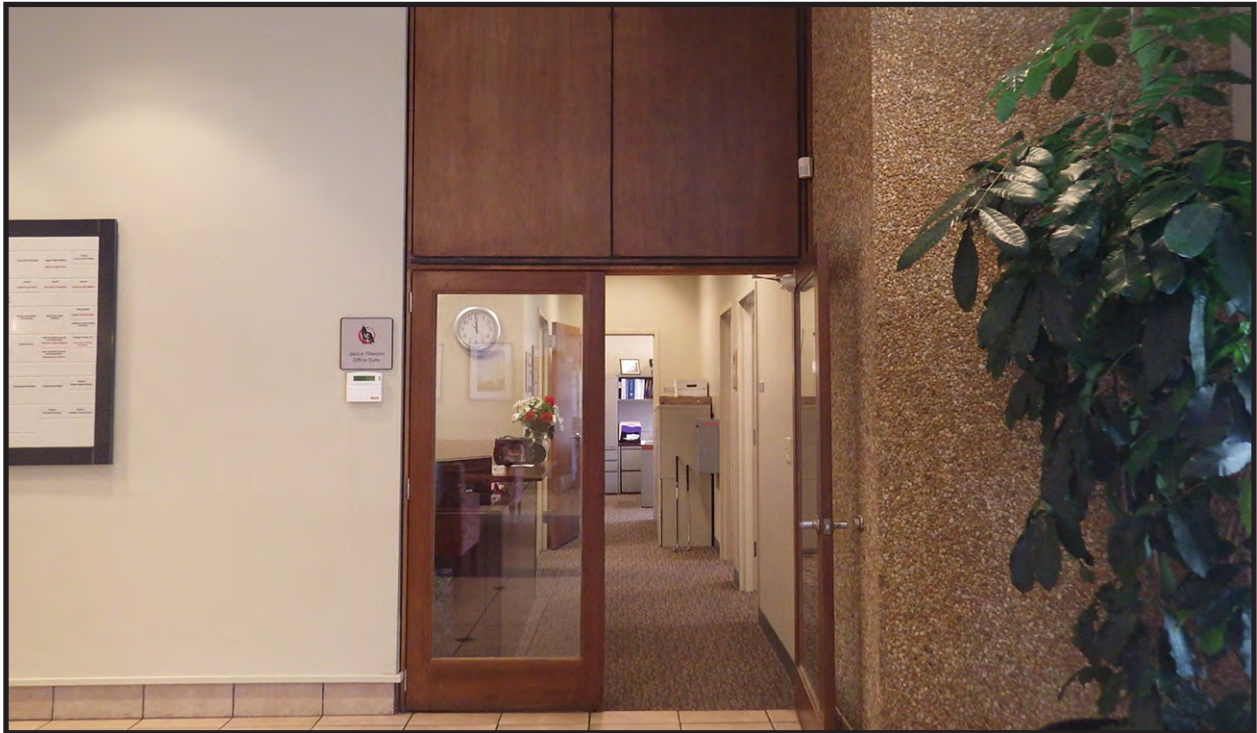
Figure 81. View from Reception Hall to Staff Offices Showing Original Pebble Dash Wall Treatment, New Paneling, Drywall, Drop Ceilings and Floor Tile
